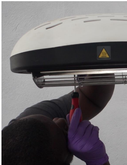
7.16 Use a screwdriver to open the heater housing.
