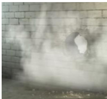
5.2 Damage from a pressurised oxygen cylinder breaking through a cement wall.
